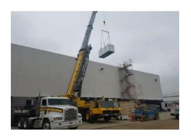
With proper preparation at the job site a two and one half hour installation per unit is achievable
